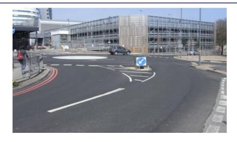
Complete reconstruction of two of the main traffic junctions into the hospital complex as part of the redevelopment of the Queen Elizabeth Hospital. The junctions, A & B, were re-constructed on a phased basis to suit programming requirements of the new Hospital project.
